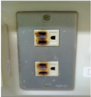
Burned out electrical outlets
