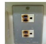
▲Burned outside of outlet
