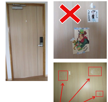
Scratches on door surface
