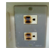
▲Burned outside of outlet
